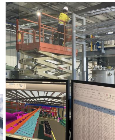
View looking out to the warehouse from the control centre
